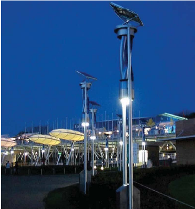
Figure 24: The use of multiple hybrid systems not only improves power output but also system cost by allowing the systems to share electronic componentry.
