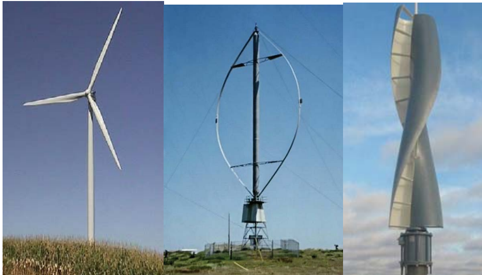
Figure 10: Wind turbine schemes: A) Horizontal axis wind turbine [6] B) Darrieus wind turbine [7] C) Helical Savonius wind turbine [8]
