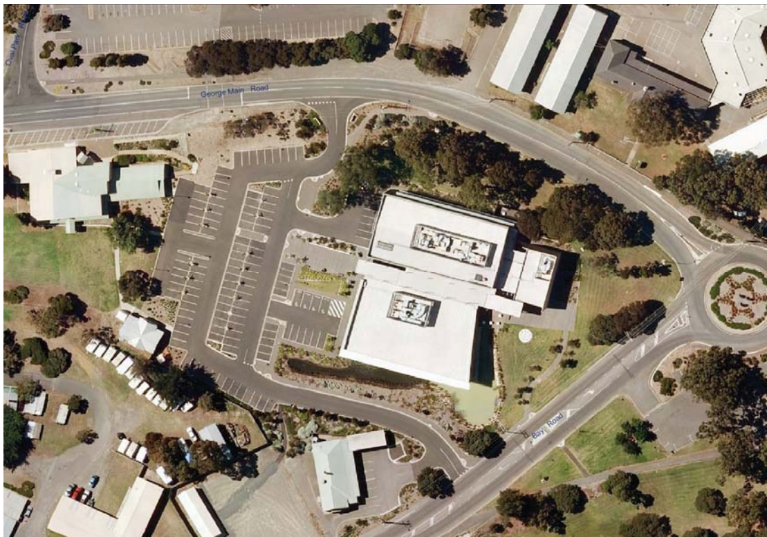
Figure 4: The Victor Harbor City Council Civic Centre - test site for the hybrid system concept.
